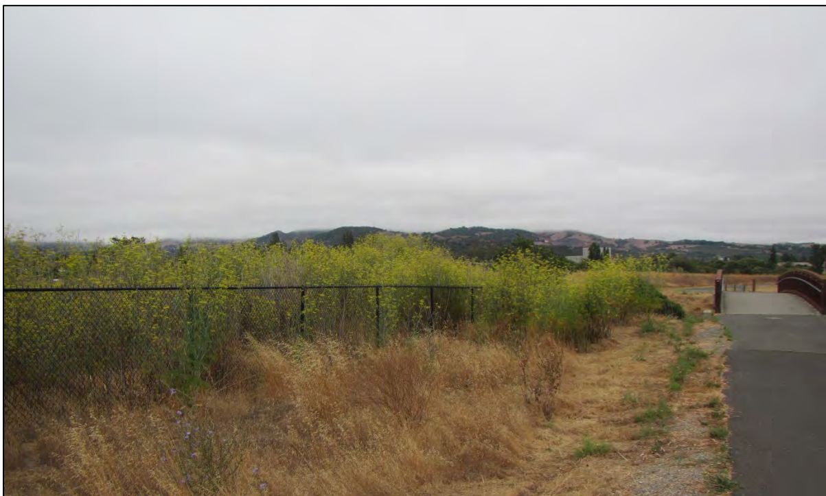
Figure 5-1: Inspection Point NLT3_2020_0012: Fence along the levee toe.
